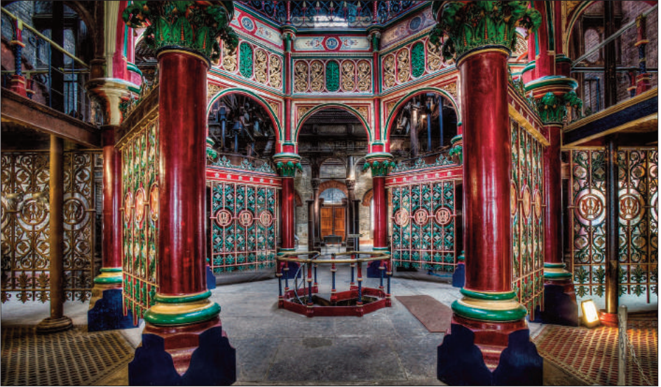
The pumping station at Crossness was opened in 1865.
