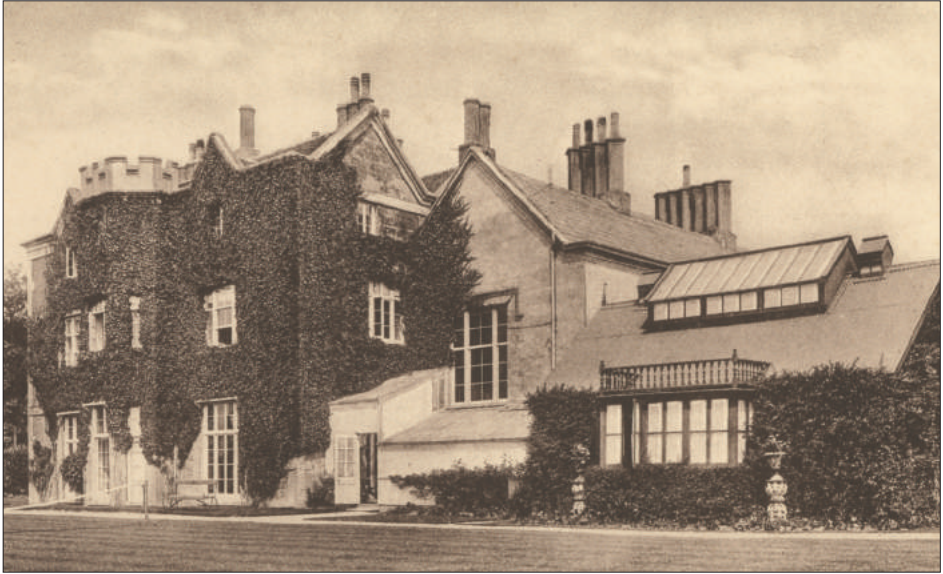
Photograph of Withersdane Hall showing Dean Crake's new billiard room.
