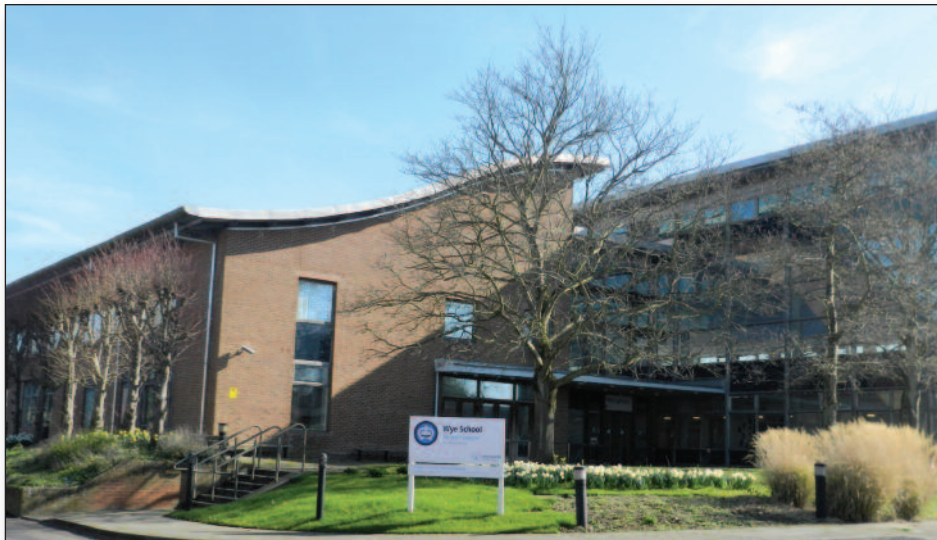
The new Wye Free School that opened in 2013 with a complement of 60 pupils. The Kempe Centre has been transformed into classrooms and an indoor gym.
