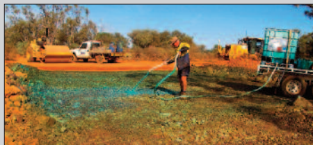
A Stonewall-treated rock chute installed to stabilise the erosion gullyhead on the Monler/Mount Margaret boundary
