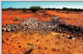
Rock-chute installed in Zoe's Gully and stabilised with GeoSpray (see above)
